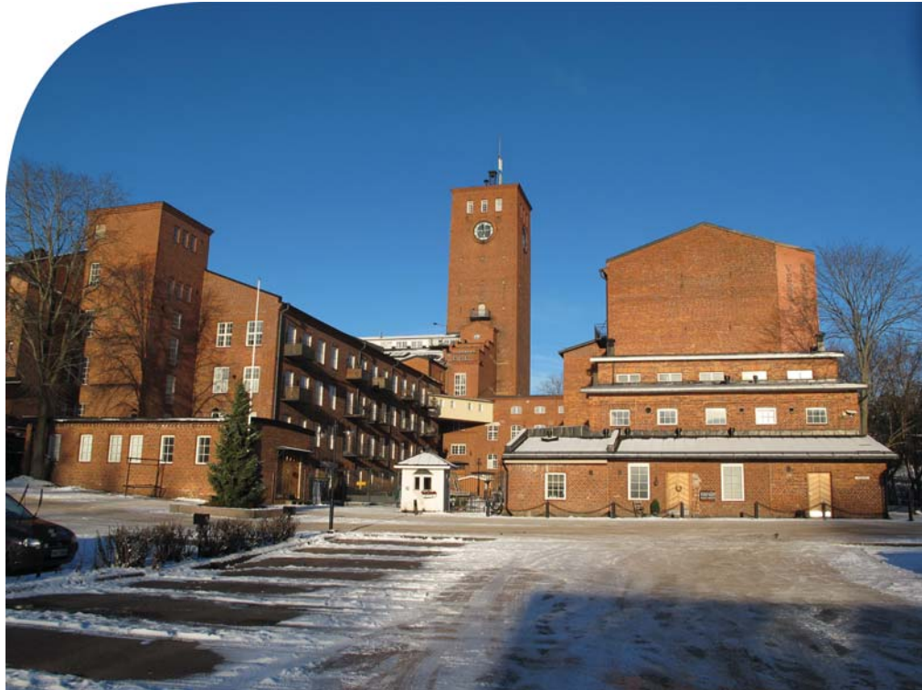
The old Littoinen cotton mill area has been converted to attractive housing area.
